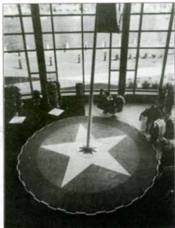
The floor of the Armel-Leftwich visitor center at the U.S. Naval Academy. The linoleum flooring was cut with high definition water jet cutting. Note the constellations.
