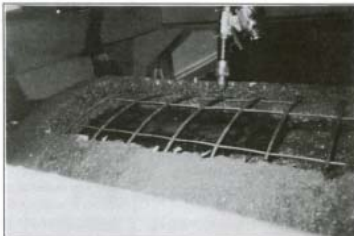
Hydrodemolished concrete on pipe cutting accomplished under water.
