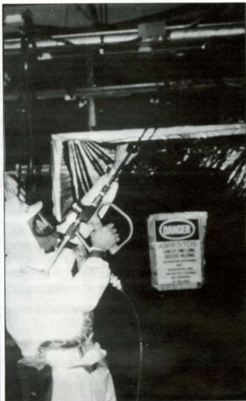
Asbestos worker using a servojet water jetting tool to remove asbestos.
