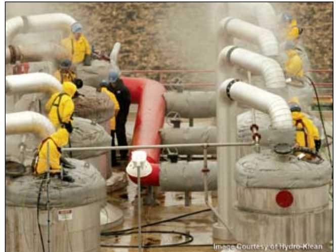
Technicians use waterblasting equipment to clean evaporator tubes at an ethanol plant. Cleaning shutdowns at ethanol plants require expert planning, communication, and execution to return the plant to full production without delay.
