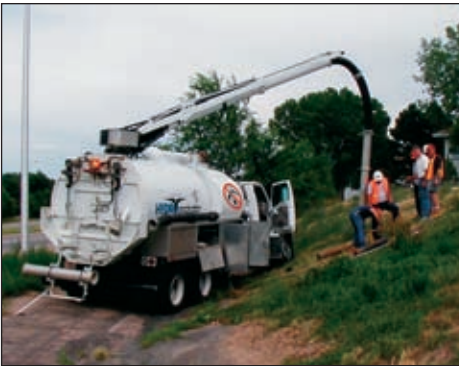
Water Shutoff Repair
