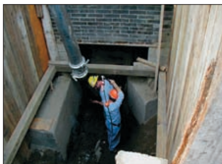
Repairing Steam Line Under Foundations
