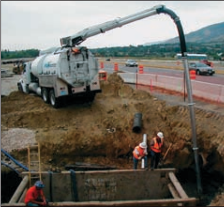
Drilling Mud Removal
