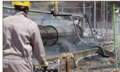
Baker helps Jetstream's customers identify appropriate hands-free waterblasting solutions, such as bundle cleaning systems for cleaning heat exchangers, evaporators, condensers and similar tube bundles.
