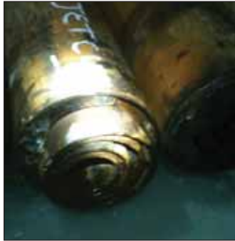
Four layers of casing were jet cut six inches below the surface casing at 30.5 feet.
