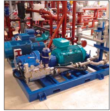
Hughes HPS3000 pumpset installed.
