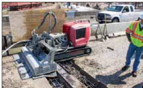
Jetstream has partnered with manufacturers, like Aquajet Systems, to offer customers category-leading specialty equipment, automated and robotic tools and accessories. The Aquajet Cutter 710 robot is ideal for hydrodemolition work on roads, bridges and runways.
