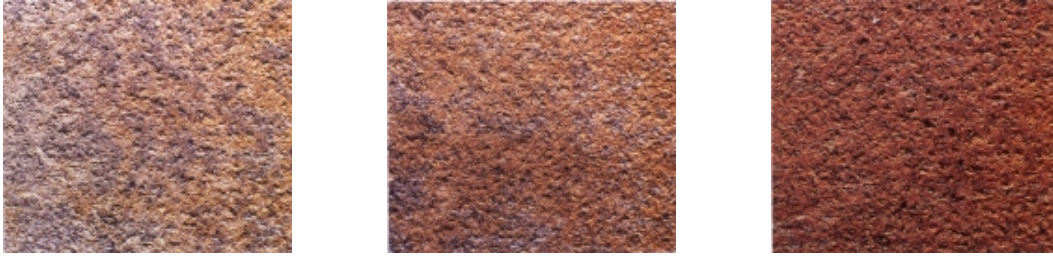
Figure 4 Examples of Light, Moderate, and Heavy Flash Rust from REF 1
