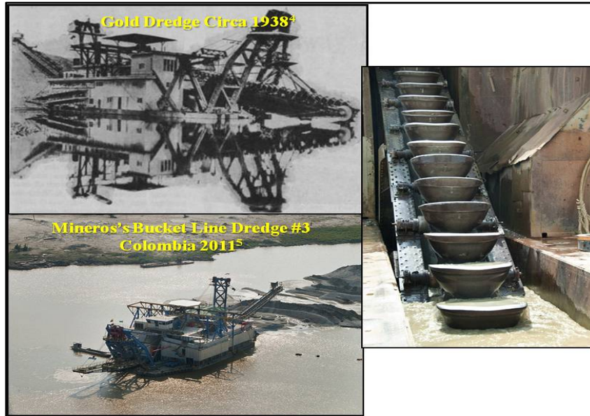
Figure 4. Bucket Line Dredges Then and Now 4,5
