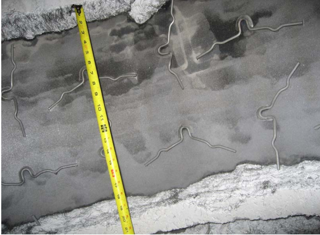
Results of Waterjet Removal in Type 1 Refractory, 1 Hour Duration Figure 2.
