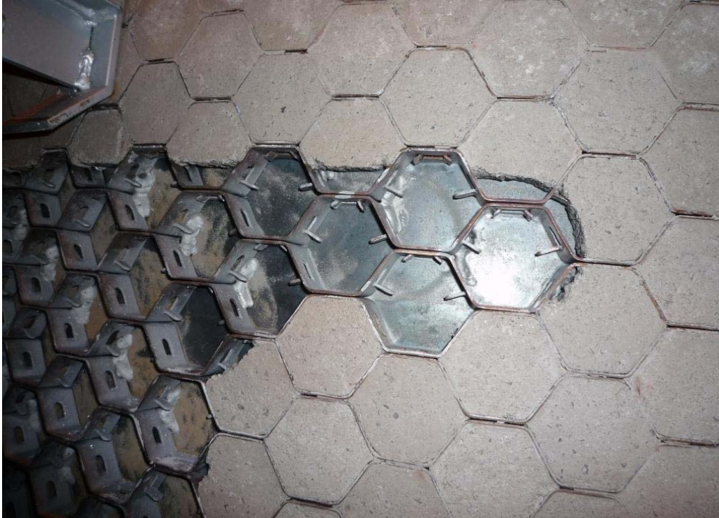
Complete Removal by 2-D in AA-22 Refractory Figure 8.
