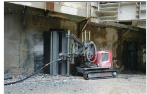
Vertical removal under the box beams.
