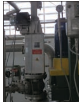
Cleaning System on Plant
