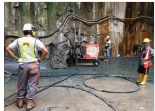
Patch removal on the floor.
