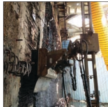
Continuing the operation up to 7 meter vertically.
