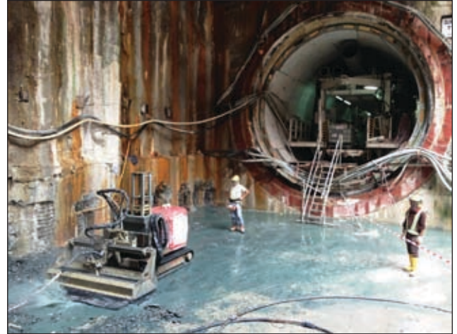
The 710V robot processes the floor in front of train tunnel.
