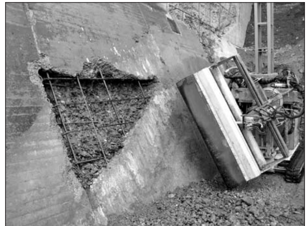
Evolution robot removing a triangle part of the cracked concrete.
