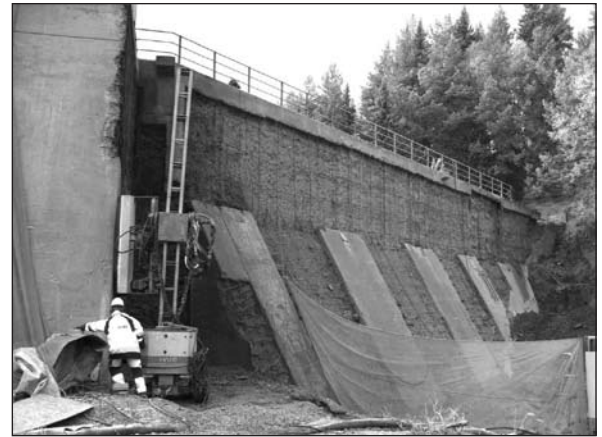
The downstream damside ready for new concrete.
