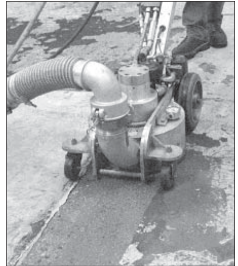
Semi-automated tools are the most popular for performing coating removal from concrete.
